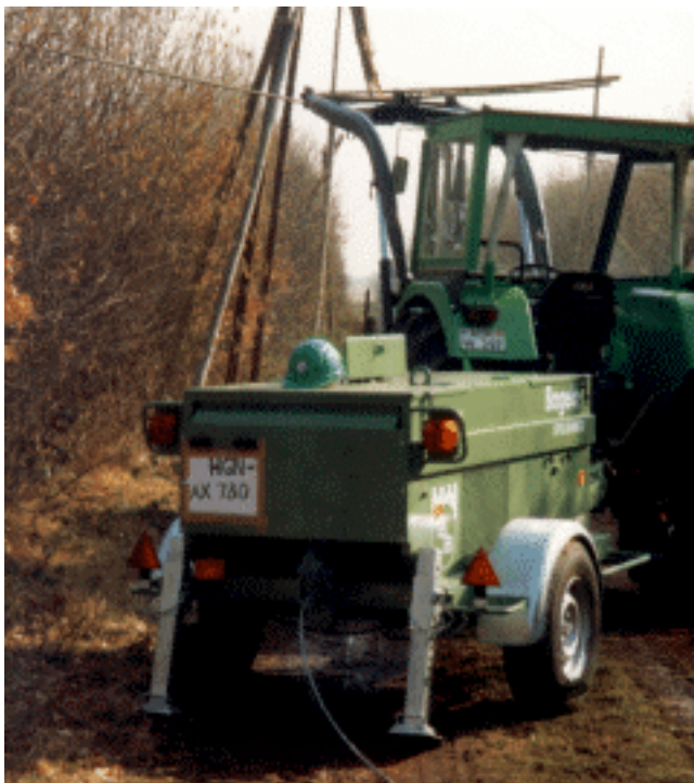
Winch KW 3F at dismantling job on a 110 kV overhead-line
